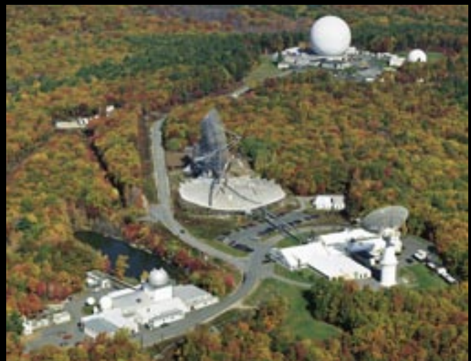
▲ Haystack Observatory facilities occupy wooded hills in northeastern Massachusetts. Shown in the photograph are the Haystack 37-meter radio telescope and radar in the large radome (top right), the Millstone Hill incoherent scatter radar antennas (center), the Lincoln Laboratory Millstone Satellite Tracking radar 26-meter antenna (bottom right), and the Firepond optical facility with its 1.2-meter telescope (bottom left).
