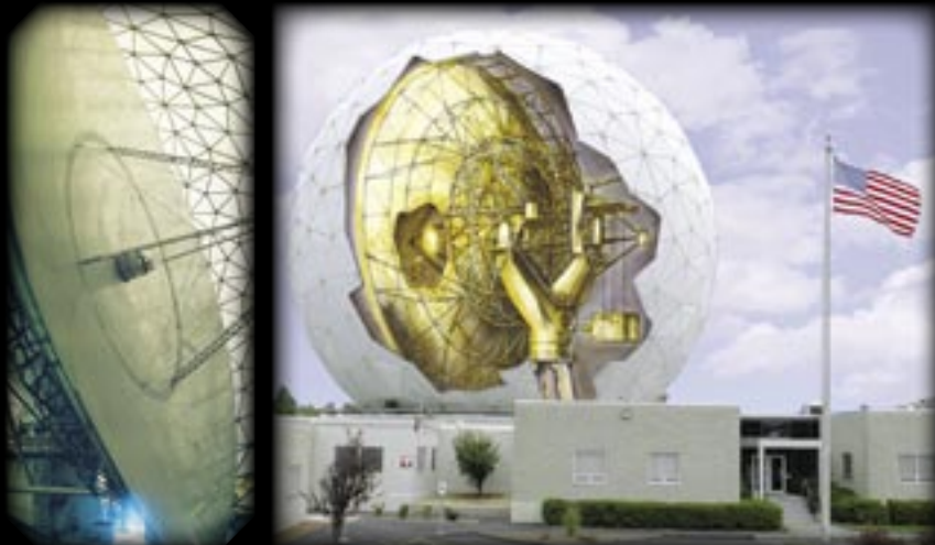
▲ Haystack 37-meter radio telescope with a cutaway view of it in its radome.
